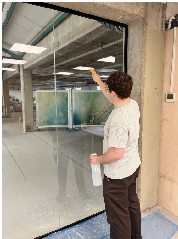
2.3.5. Wipe the glass with isopropyl alcohol and a new, unused lint-free cloth
